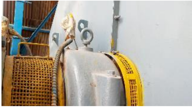
RTD for Bearing Temperature
